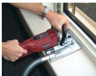
Cut into the window frame
