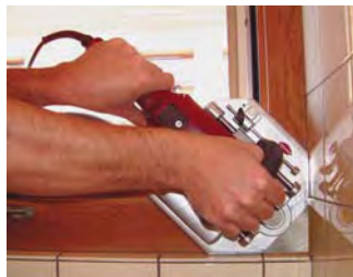
Cut into the wall
