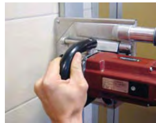
Cut into the tiled wall
