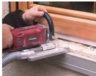
Cut-out for the weatherboard
