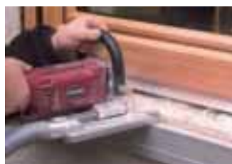
Cut-out for the weatherboard
