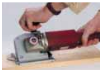
Planing protruding patch
