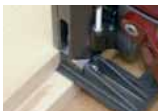
Repair in the groove
