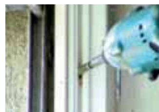
4. Install the new window
