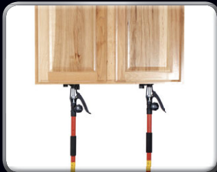
Installing cabinets
